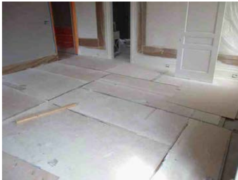
Bedroom Unfinished Work
